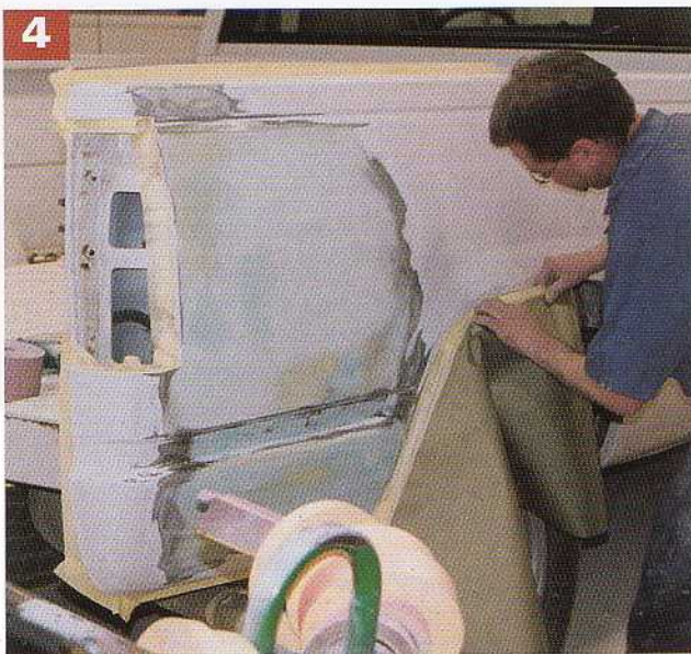
4 Masking paper is then taped into place along the wheelwell to cover the wheel, tire, and inner fender.
