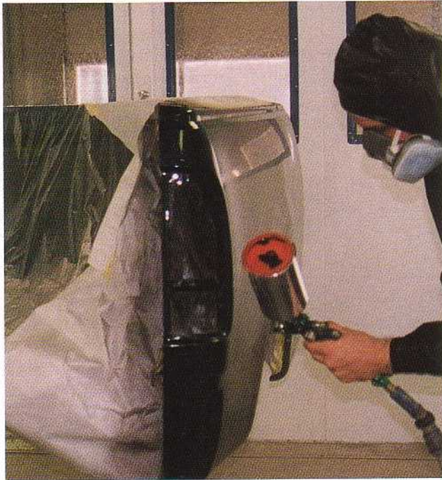
Even when painting the subtle wheelwell flare, position the spray paint gun so that it is perpendicular to the area that bulges slightly from the main panel. The flare varies in width from about 1 inch to about 2 inches wide, so it is not a large area, however, it is still important to apply the paint evenly. Remember that when using a base coat/clear coat paint system, the base coat should be applied only to achieve complete coverage. Gloss will come from the clear.
