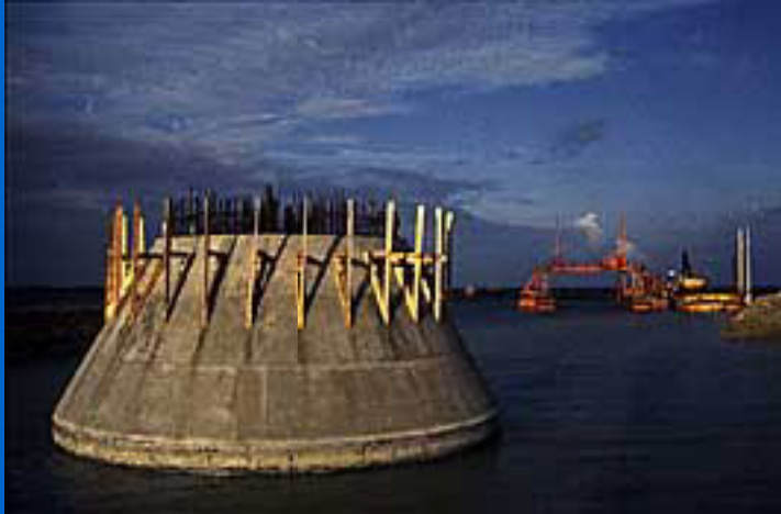
Foundation being floated out to Tunoe Knob Photograph © 1996 by Flemming Hagensen
